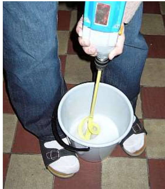
mixing the silicone resin components
