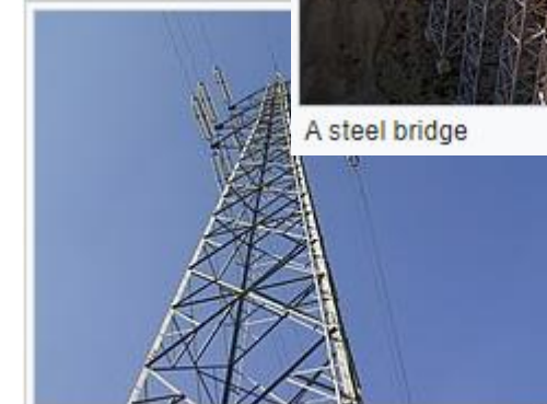
A steel pylon suspending overhead power lines
