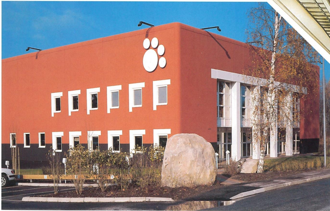
Saddle TT-roof slabs on load-bearing sandwich walls
