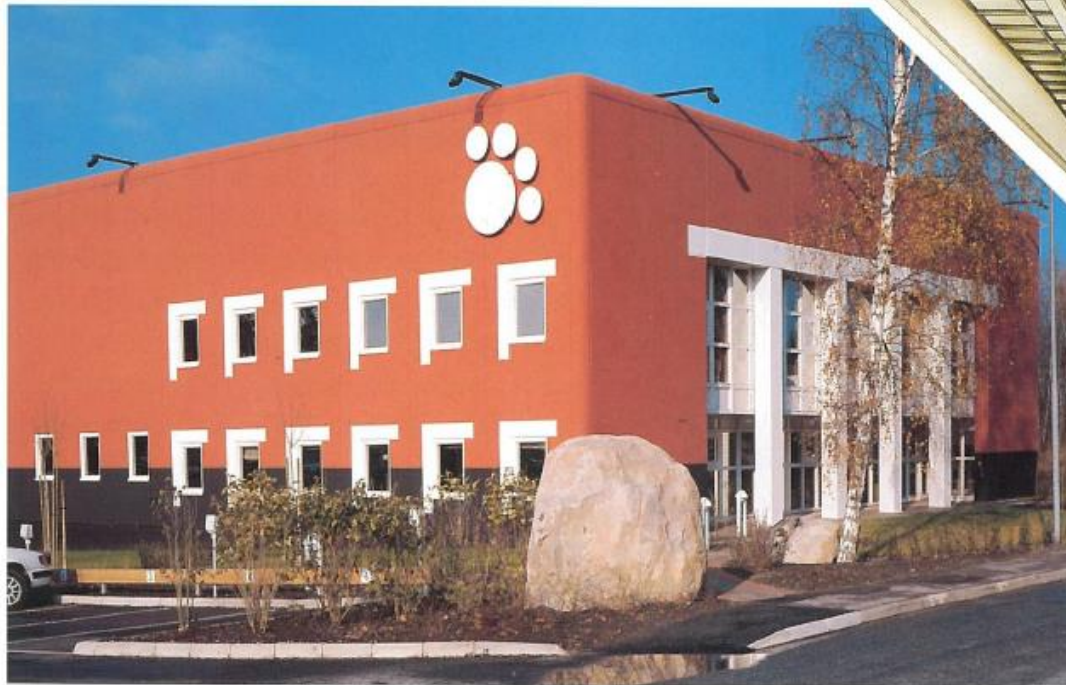
Saddle TT-roof slabs on load-bearing sandwich walls
