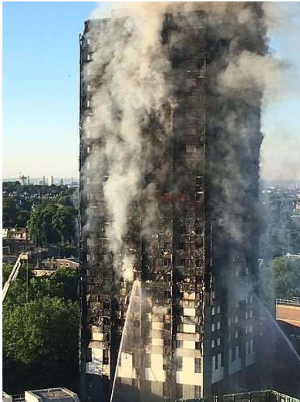
Obr. 2 Požár Grenfell Tower [2]
